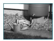
**6** Use: After a rainfall, fill a watering can using the bottom spigot or attach a hose to use the water where it's needed.
