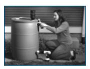
Overflow: Drill a hole near the top of the barrel to accommodate an overflow pipe that is at least 2 inches in diameter. If the overflow pipe elbow seals and seats securely, it can be threaded directly into the barrel opening. If not, it should be secured with washers on both sides of the barrel and a nut on the inside. Use Teflon tape around the threads and a bead of silicon caulking around the opening to ensure a tight seal.
