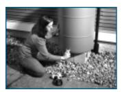
Outlet: Drill a hole near the bottom of the empty barrel to attach the drain spigot. If the spigot seals and seats securely, it can be threaded directly into the barrel opening. If not, it should be secured with washers on both sides of the barrel and a nut on the inside. Use Teflon tape around the threads and a bead of silicon caulking around the opening to ensure a tight seal.
